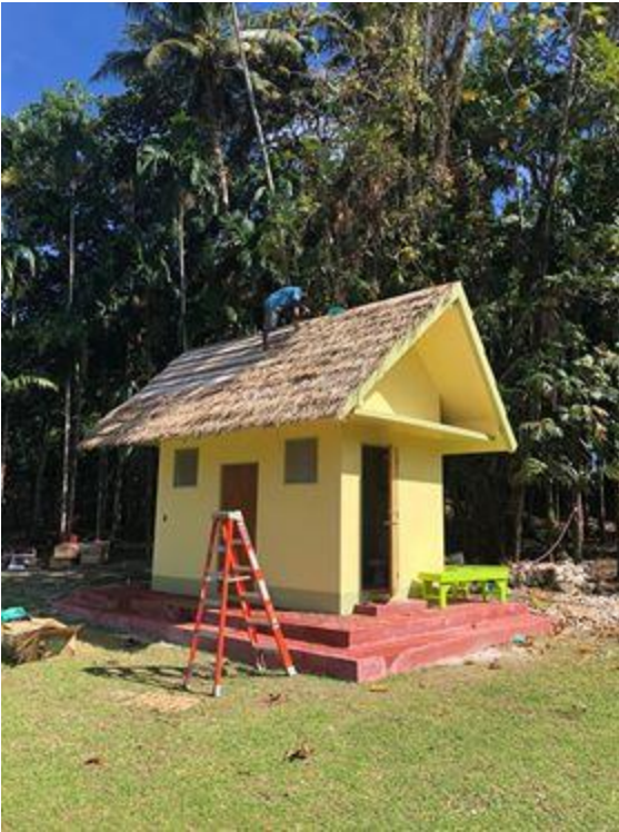
New Restroom facilities next to Airai Bai
